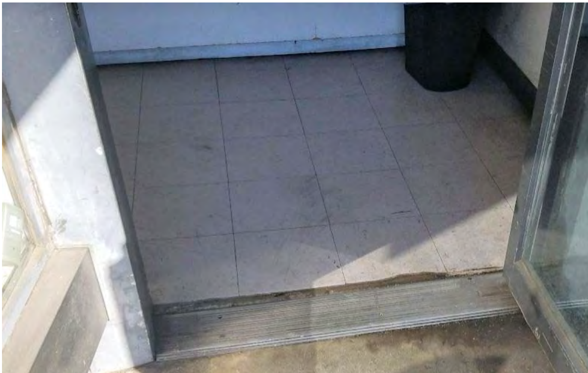
Area OF 12' x 12' Floor Tiles Southwest Side Of Property
