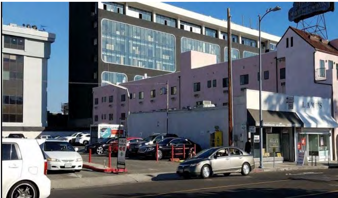
South Side Of Property
