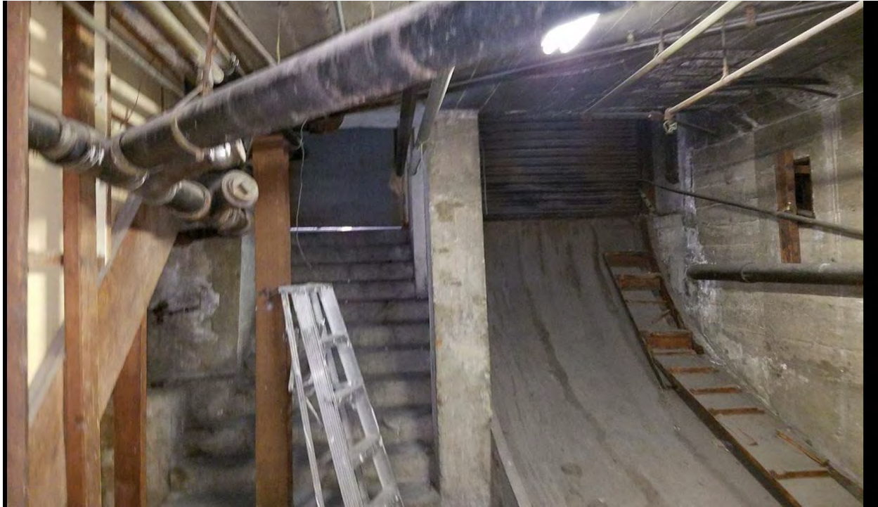
Ramp From Inside To Slide Goods Into South Basement
